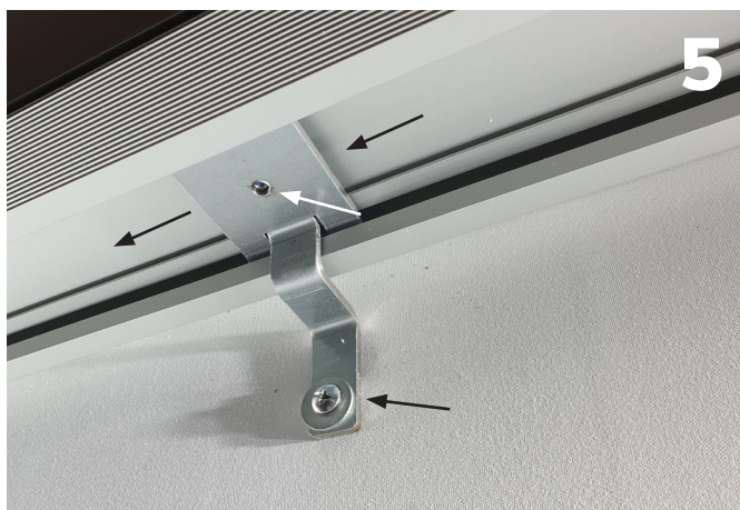
Insert the wall bracket into the groove of the profile, tighten the stabilizing thread and fasten it to the wall directly through the already inserted rear unprinted canvas.
